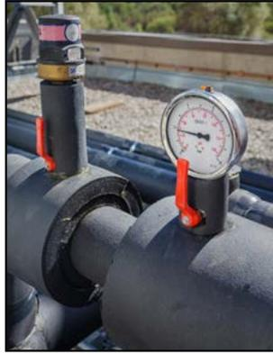
and installed system should be sized correctly so it does not compress the insulation. See “Cladding | Jacketing” schedule under Technical Resources for AEROFLEX pipe insulation OD’s.
