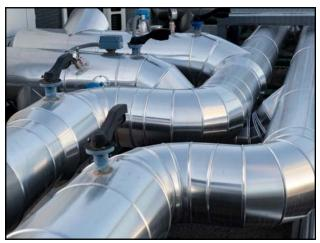
Aeroflex USA does not recommend specific protective jacketing systems. However, the specified and installed system should be sized correctly so it does not compress the insulation. See "Cladding | Jacketing" schedule under Technical Resources for AEROFLEX pipe insulation OD's.
